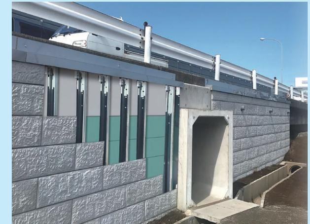
Foam-support construction method registered with NETIS.
