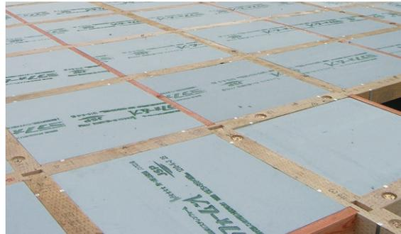
Pre-cut thermal insulation material MIRAFOAM (lambda)
